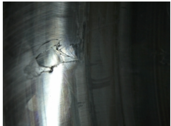
Figure 5 – Outer race damage found at front side bearing
